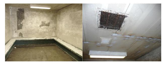
In one of the larger cells a deputy explained that the thermostat control for the cell was located above the vent in the cell. It is apparently accessed through a crawlspace from an access door about sixty feet away. The thermostat is not adjusted.
