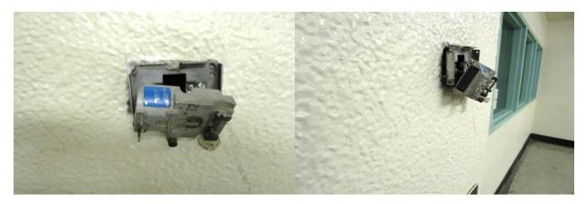
There is a climate control box on the 8th floor that is hanging off the wall. It apparently had been damaged for quite a while.
