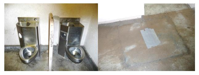
Plumbing and sewage issues are a problem with inoperable toilets and sinks. Jailers have to find ways to control the odors (such as taping over floor drains).
