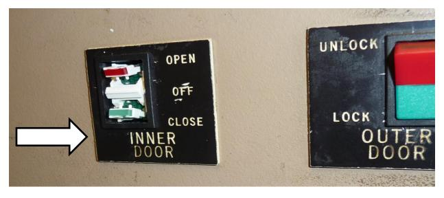
As with other courthouses, this CGJ found ongoing problems with the cell door and lock mechanisms. Switches to control either the exterior or interior doors were a problem for some of the doors. We were told that since the parts are so old they need to be specially constructed, some lock control mechanisms had to be cannibalized from locks in other areas of the courthouse. The photograph illustrates a switch that needs to be manipulated with keys, the tips of pens, or paperclips.
