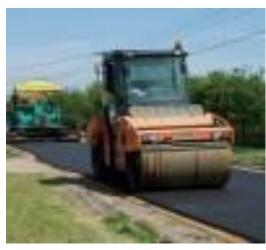
Steam Roller is the most efficient and complex way to repair potholes. This involves complete resurfacing of the street. http://thenewswheel.com/5-kindspothole-repair
