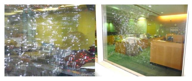
This CGJ found security windows cracked, some with heavy spider web cracks.
